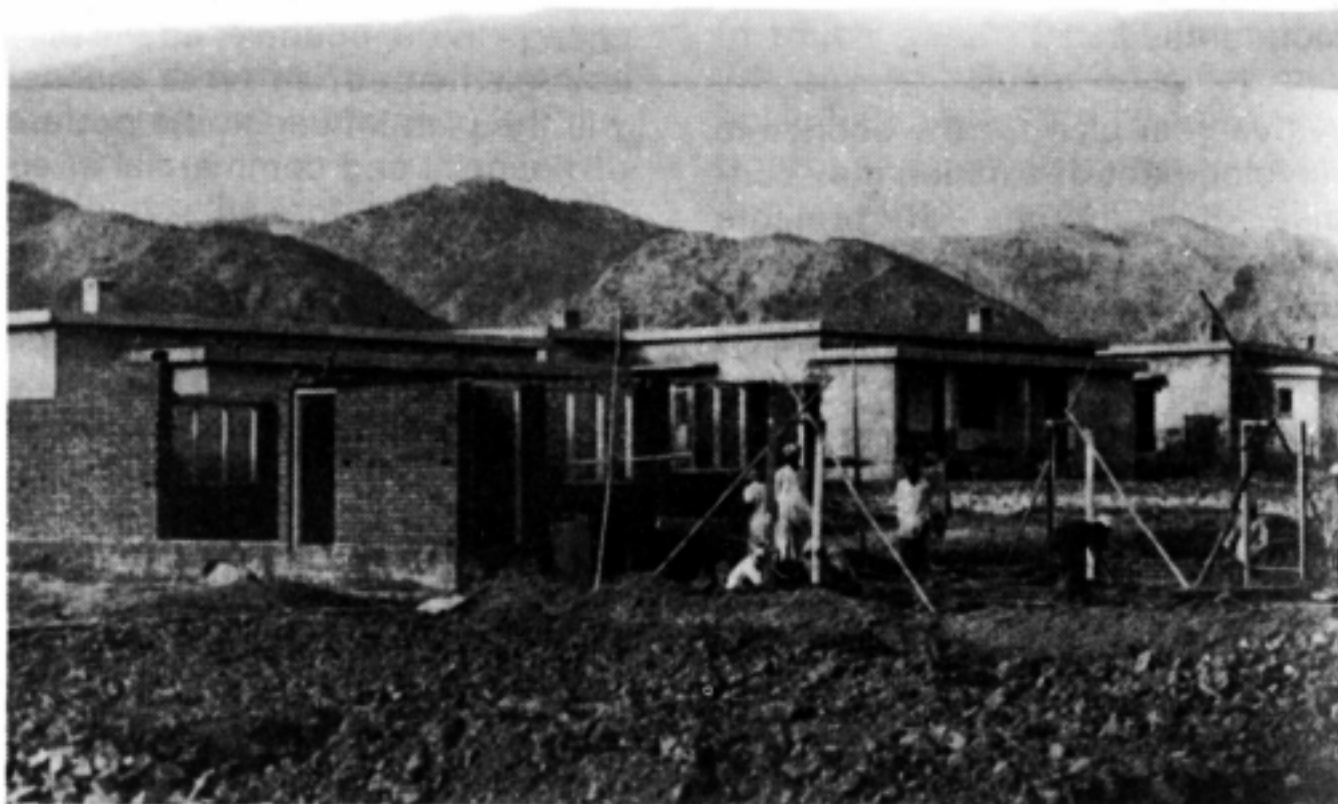
Pakistani workers constructing Islamabad, now Pakistani's permanent capital.
