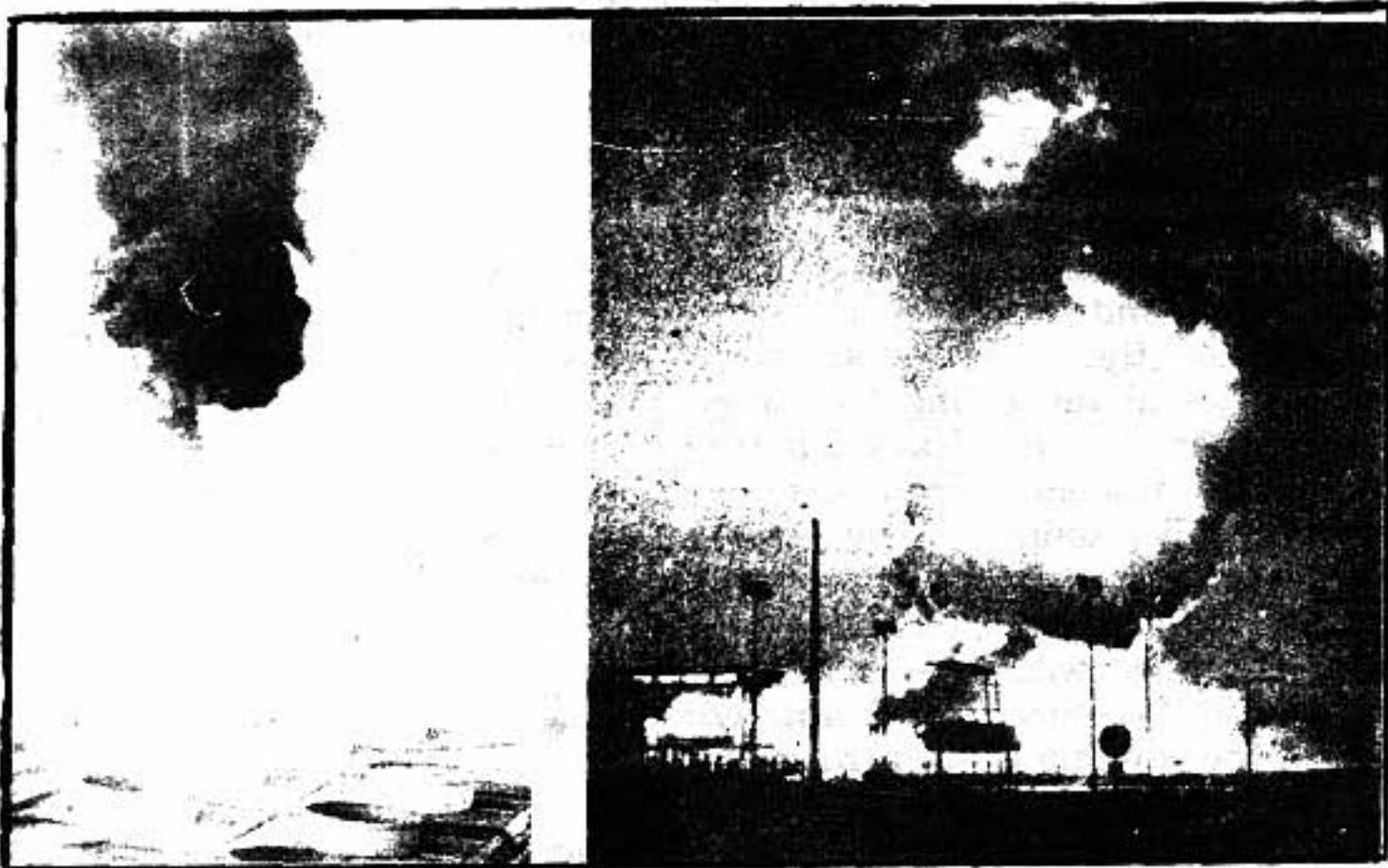
Sabotage at Sasol. Damage was to the tune of R66m
