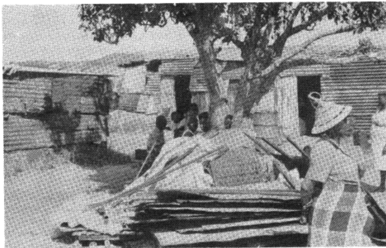
The squatter camp, with a demolished hut lying in the foreground
