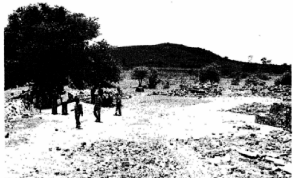
A lunch rest during the mammoth stone-cleaning operation: chipping concrete from the stones of the demolished building
