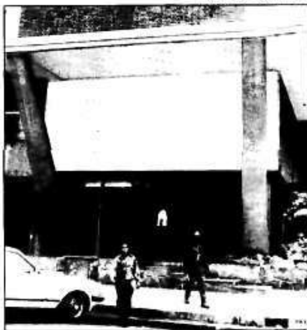
Cresthill — after intense battles, tenants are now considering buying the building.
