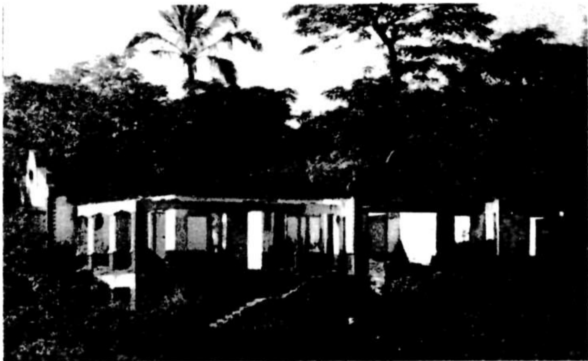
A dilapidated house bears witness to Cato Manor's troubled history
