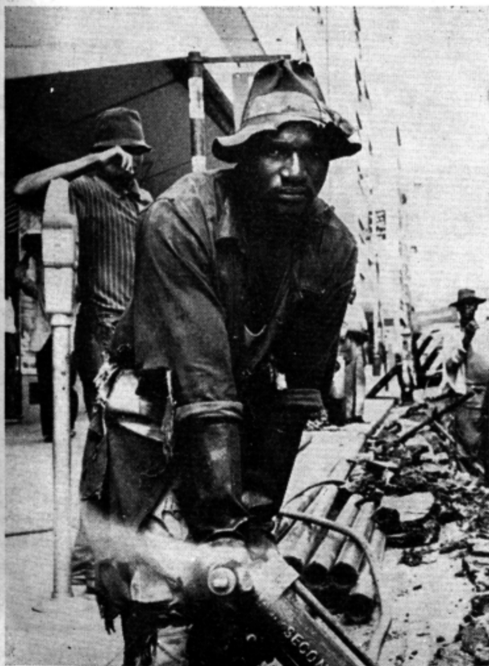
A road-digger : average wage £3 per week
