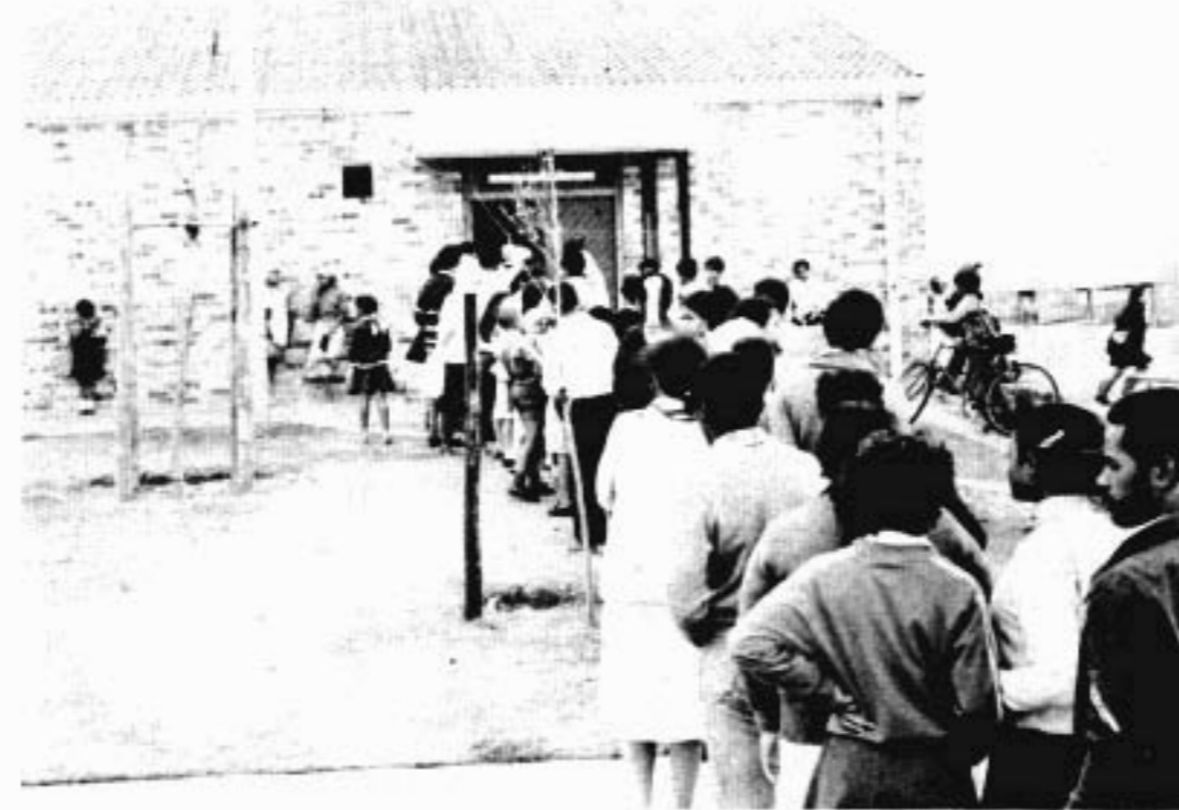
A scene at Westridge pay office on electricity due date day.
