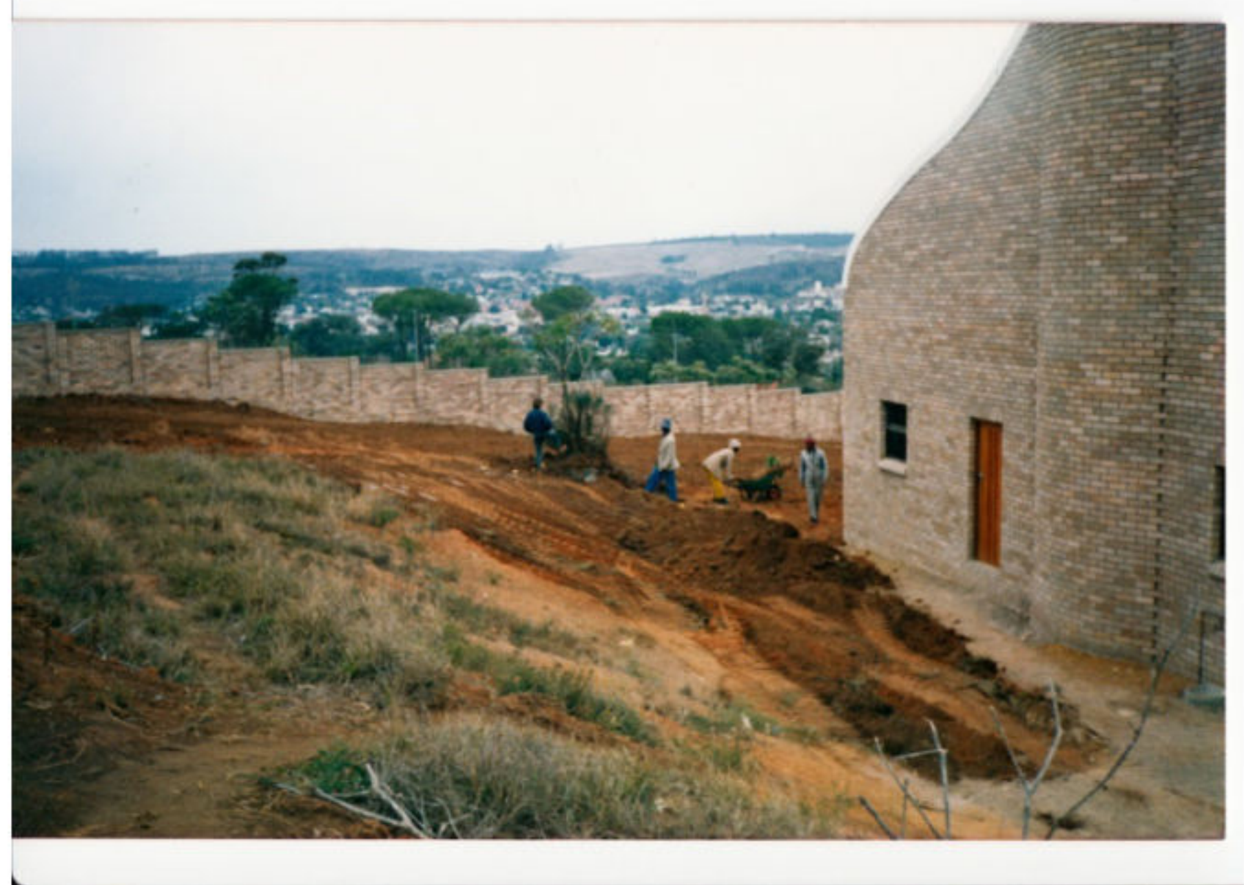
Construction of the new Mandir. Photo supplied by Mr Chiman Harjeven
