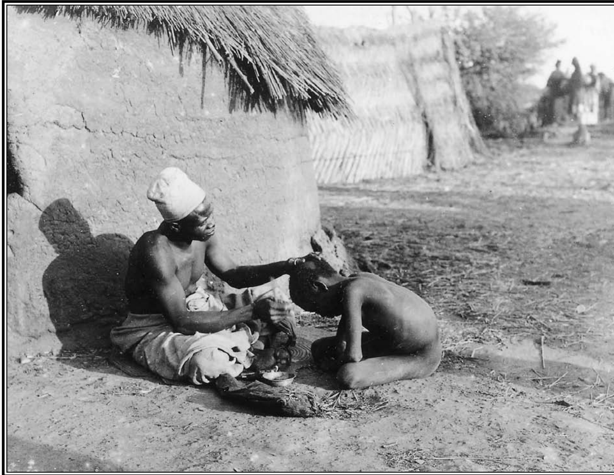
Barber Shaving Boy's Head in Front of Mud Hut, Northern Nigeria, 1898 The walls of mud huts could be as much as three feet thick. Mud huts had two serious disadvantages: they were easily eroded by rain and mud is not resistant to termites.
