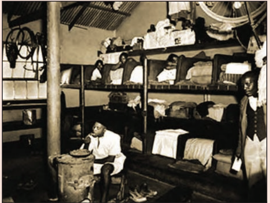
Interior of mine workers' hostel
