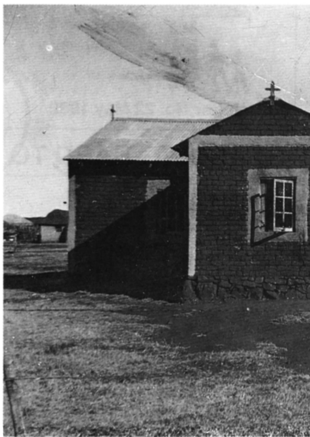
The school built by the community on their land.
