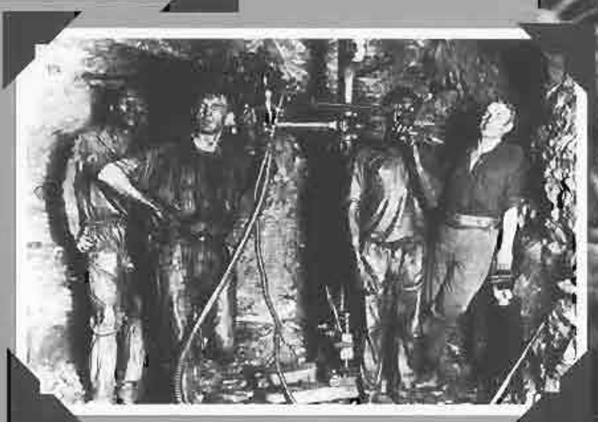
Underground workers without helmets or protective boots, 1915.
