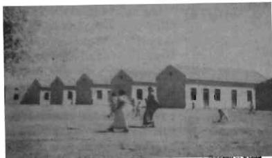
A view of some of the tenements in Kasturba Niketan, India's largest colony for displaced women, opened in New Delhi recently by President Rajendraprasad. There will be 300 residential tenements, eight huge halls, administrative buildings etc.—P.I.B.
