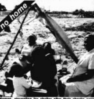
Women, struggling for shelter after their shacks were demolished in Crossroads
