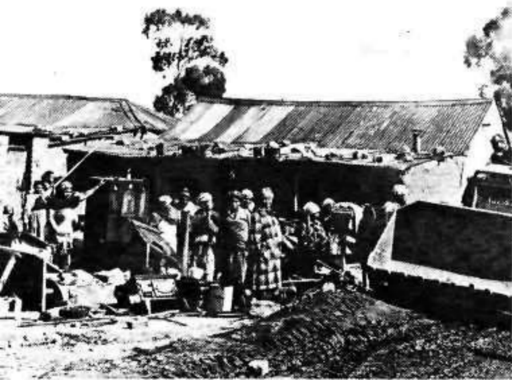
Pimville residents watch their homes being demolished
