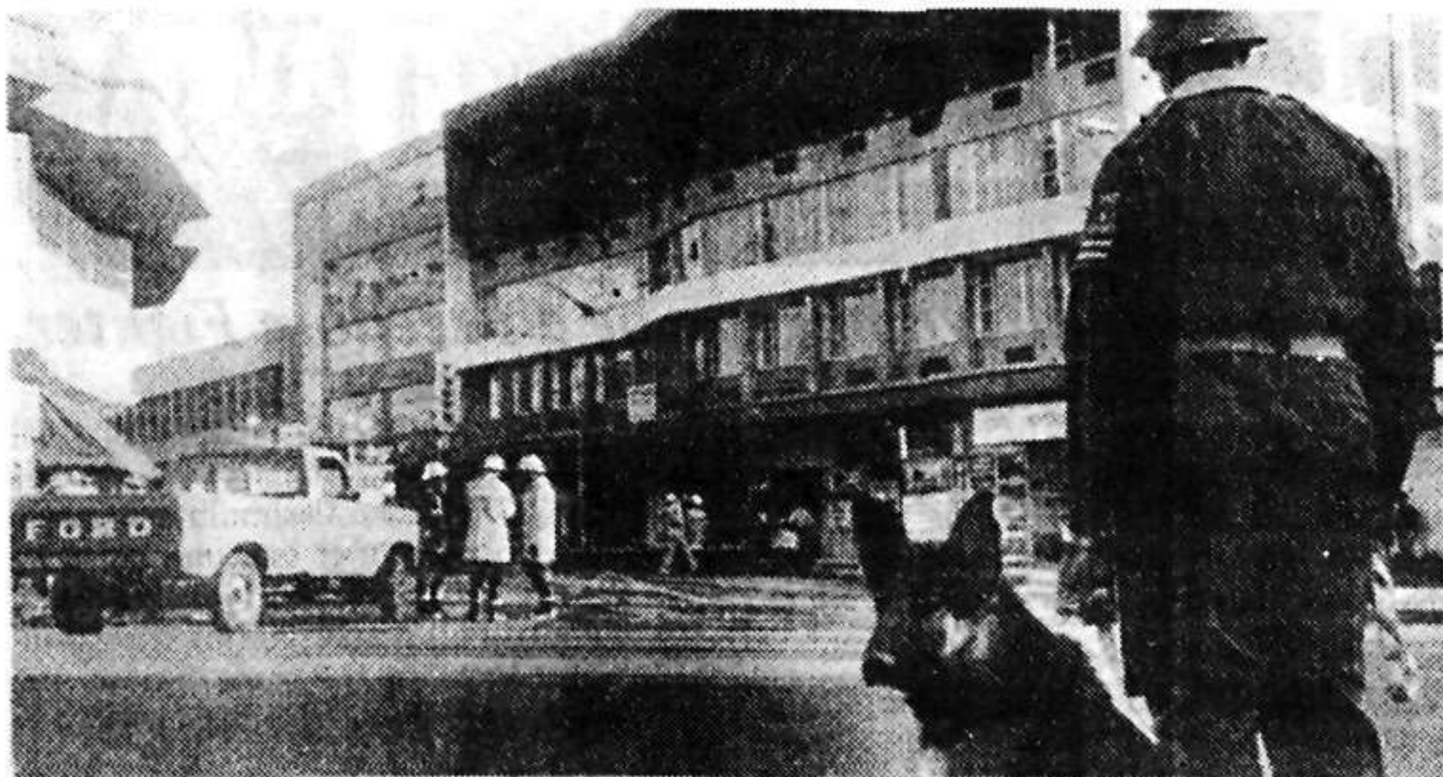
The upper storeys of the Sanlam building, Roodepoort, in flames. The building houses the Divisional Headquarters of the South African Police.
