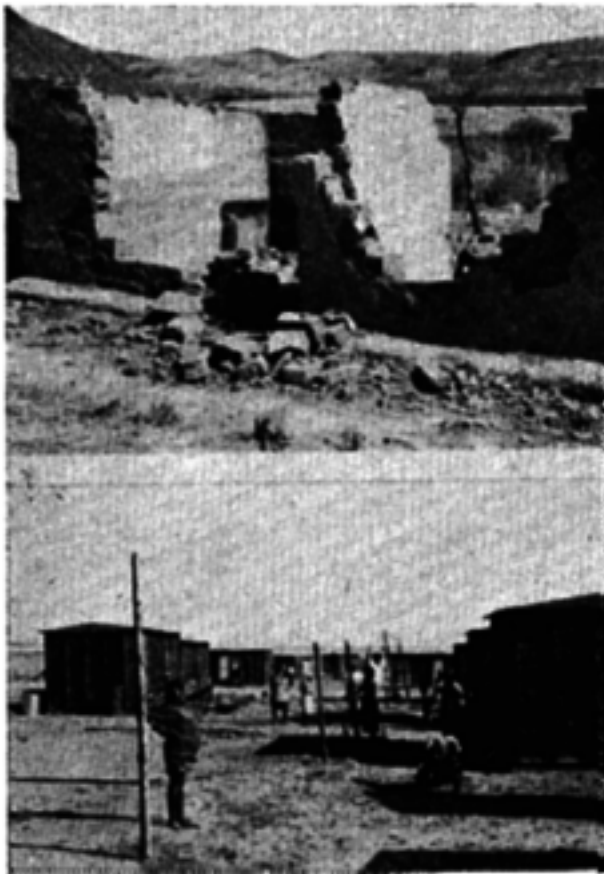
The top picture shows a section of the desolation at Charlestown. Below are the wooden huts at the Duckponds location, seven miles from Newcastle and 35 miles from Charlestown.
