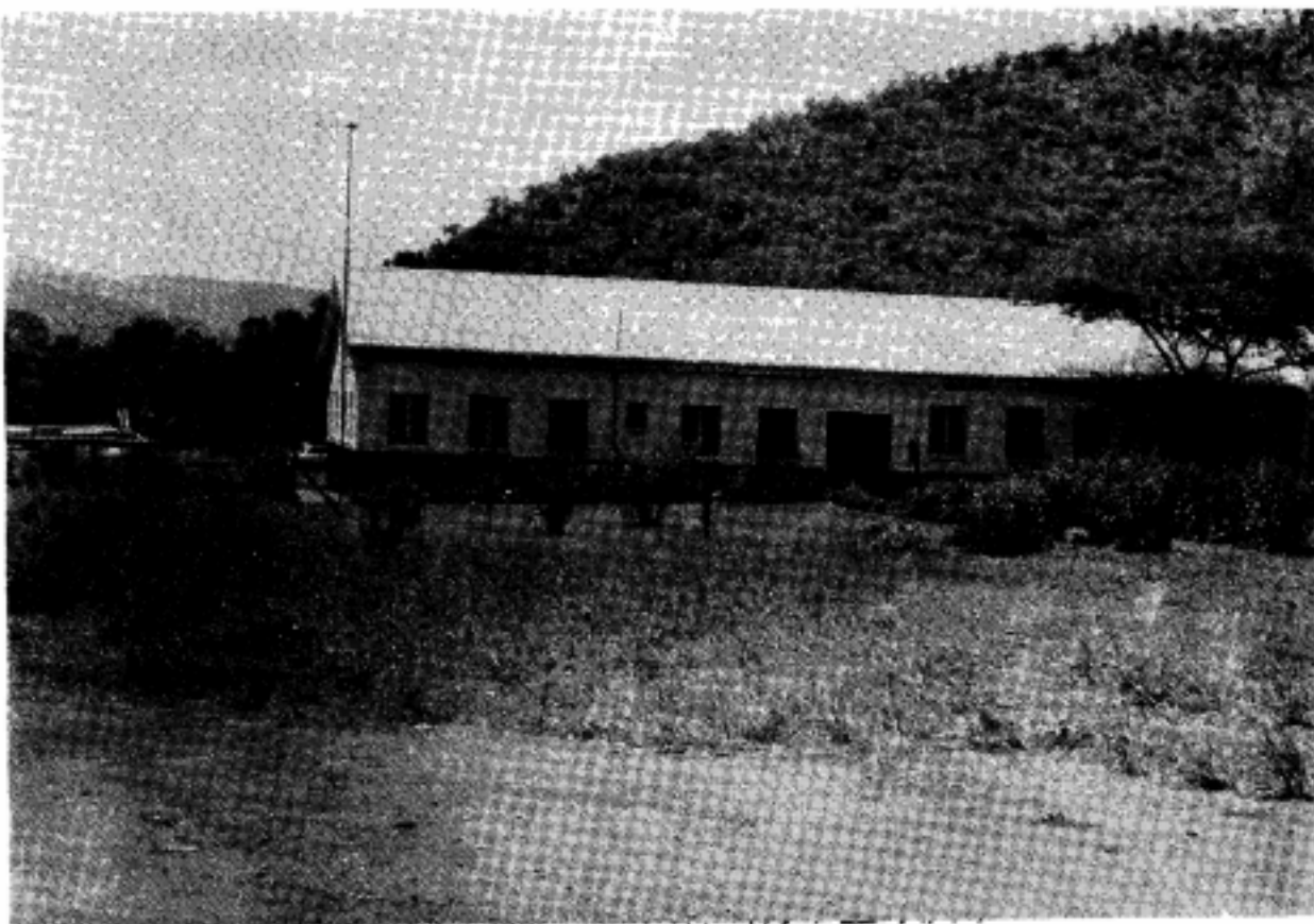
Part of KaNgwane Administration offices.
