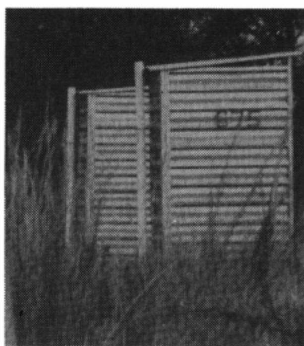
One the DDA's development projects - thousands of unused toilets.
