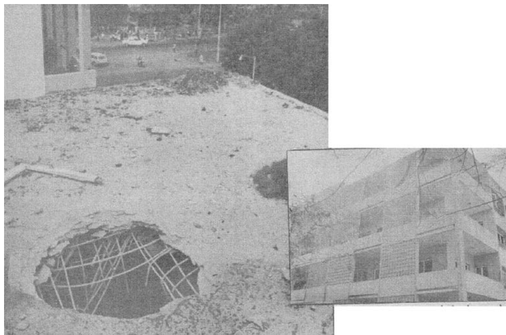
Figure 17.9: The hole caused by a bomb explosion in the building where the ANC information offices were located. Sourced from the magazine Tempo #668 of 23 October 1983
