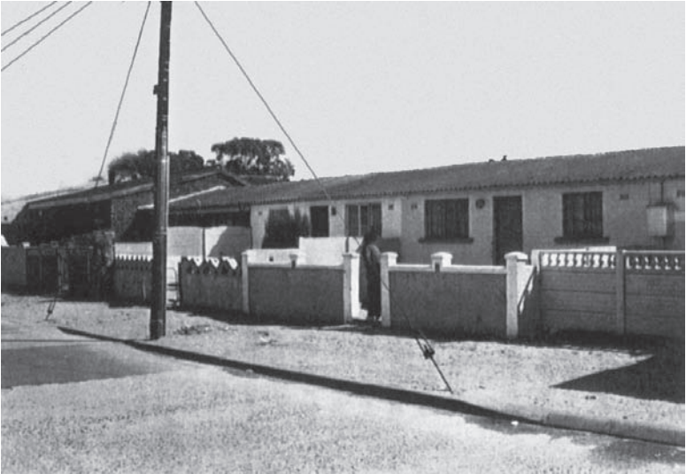
FIGURES 3.1 AND 3.2: Typical street and council houses in Guguletu township Source: Japha, Derek and Marie Huchzermeyer, 'The history of the development of townships in Cape Town, 1920–1992', The Integration and Urbanisation of Existing Townships in South Africa Working Paper no. 2 (Newcastle and Cape Town, 1995)
