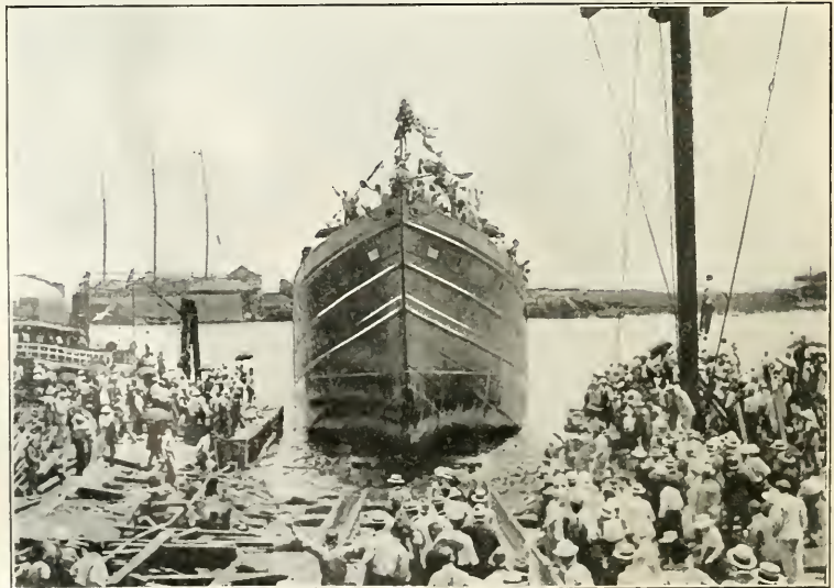
FIG. 29. — Launching a steel "Liberty Ship," shipbuilding yards, Mobile, Alabama.
