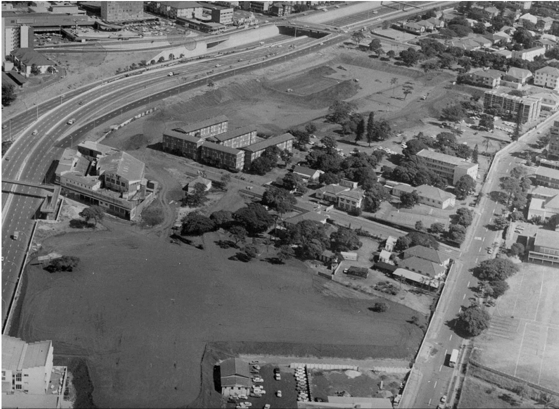
Fig 34. The site being cleared for construction of Technikon Natal in the 1980s. Some residential buildings were retained for use by the Technikon (DUT archives)
